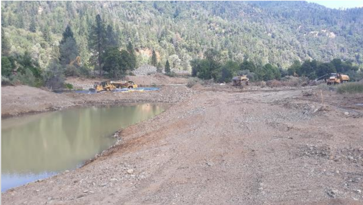
Construction of a new, longer and more sinuous mainstem Trinity River.
