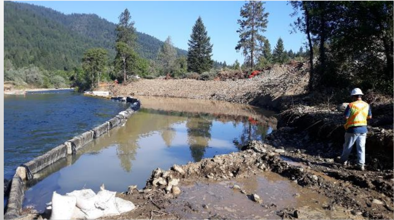
Meander construction isolated from the mainstem Trinity River. Note clear Trinity River adjacent to active work area.
