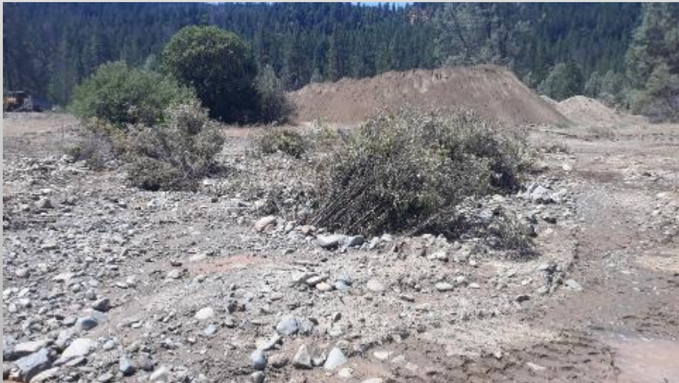
Completed willow trench plantings that will establish quickly, trap fine sediment and rapidly restore floodplain processes.
