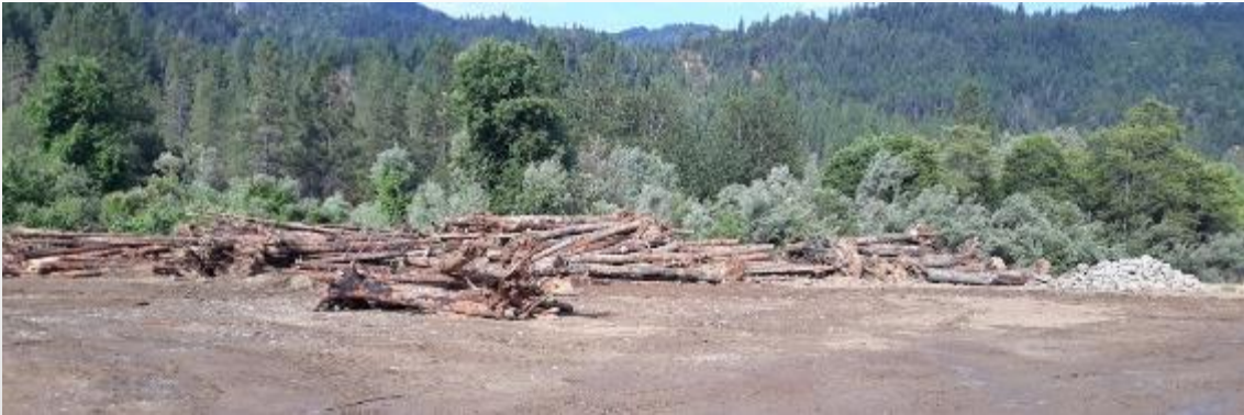
Over 500 pieces of large wood were brought to the site and used in the construction of Chapman Ranch.
