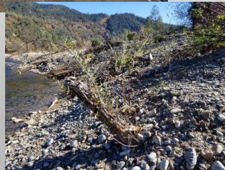
Willow clumps plated along channel margins quickly provide shade.
