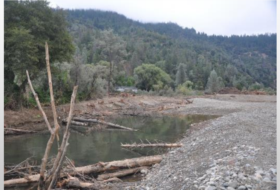
Completed alcove with large wood.
