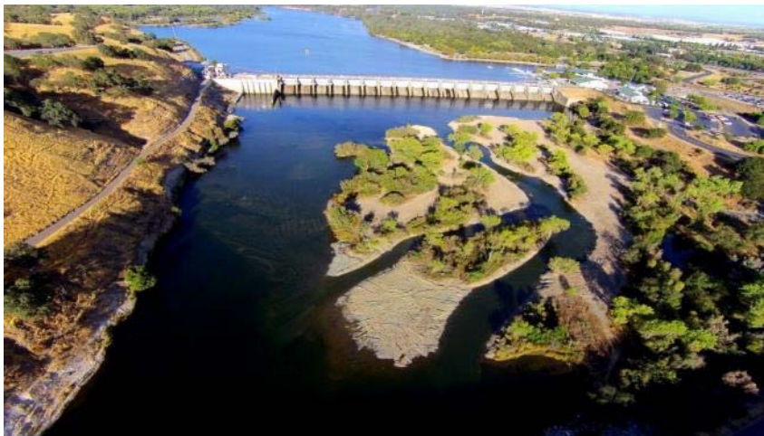
Before (top) and After (bottom) Spawning and Rearing Habitat 2014 Construction below Nimbus Dam, American River
