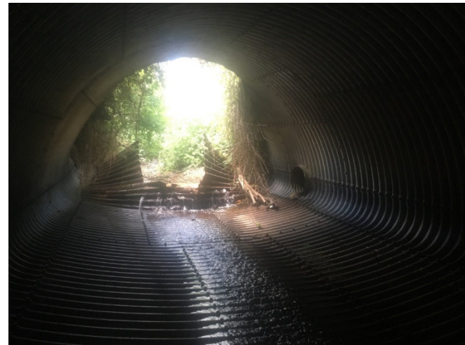
(Sydney Gulch Existing Culvert)
