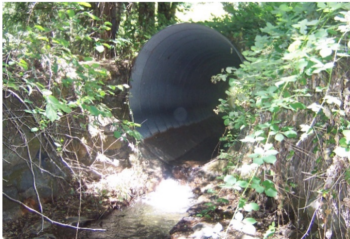
(East Branch East Weaver Existing Culvert)
