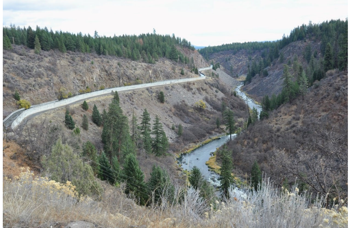
Klamath River between JC Boyle Dam and Powerhouse
