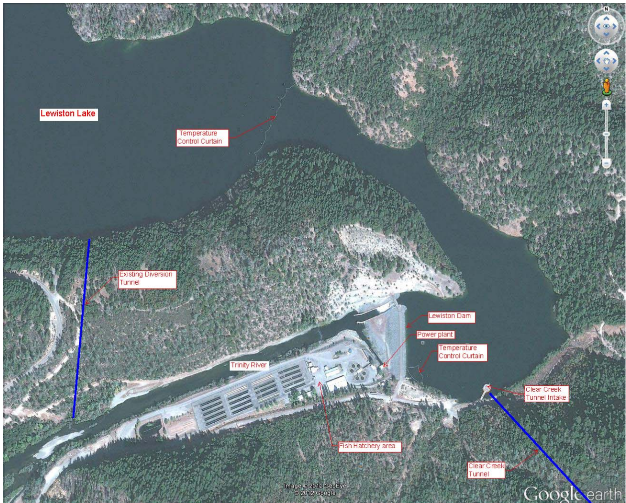
Figure 1. Lewiston Dam and Reservoir Facility and Structures.
