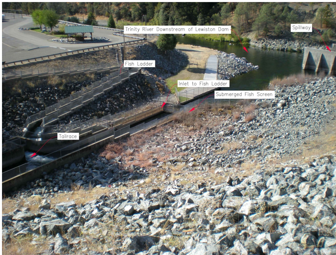
Illustration 1. Location of Fish Ladder, Tailrace and Spillway
