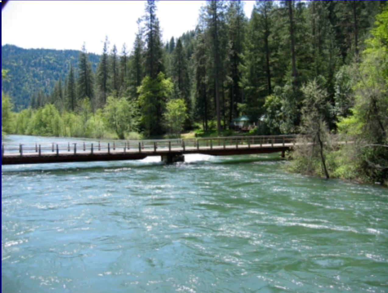
Biggers Road Bridge
