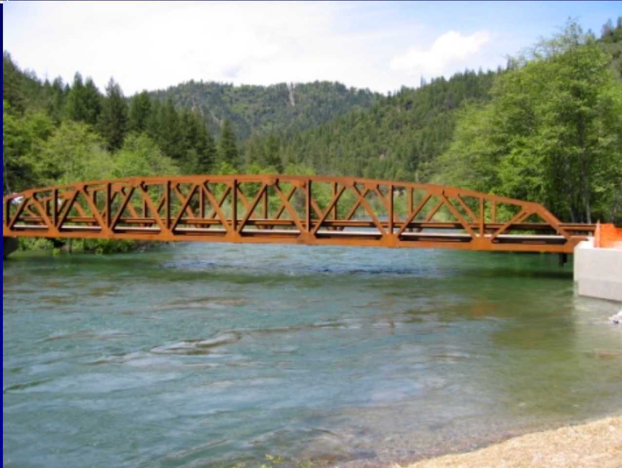
Biggers Road Bridge
