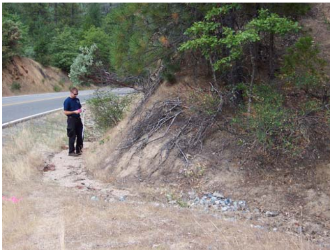
Photo C (Lower left). Trinity Dam Boulevard showing cutbank sediment delivery to a ditch.
