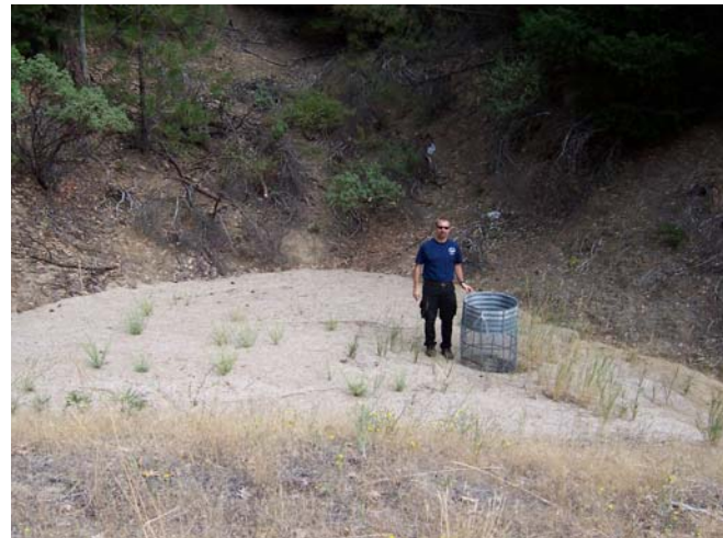
Photo C (Lower left). Trinity Dam Boulevard showing cutbank sediment delivery to a ditch.
