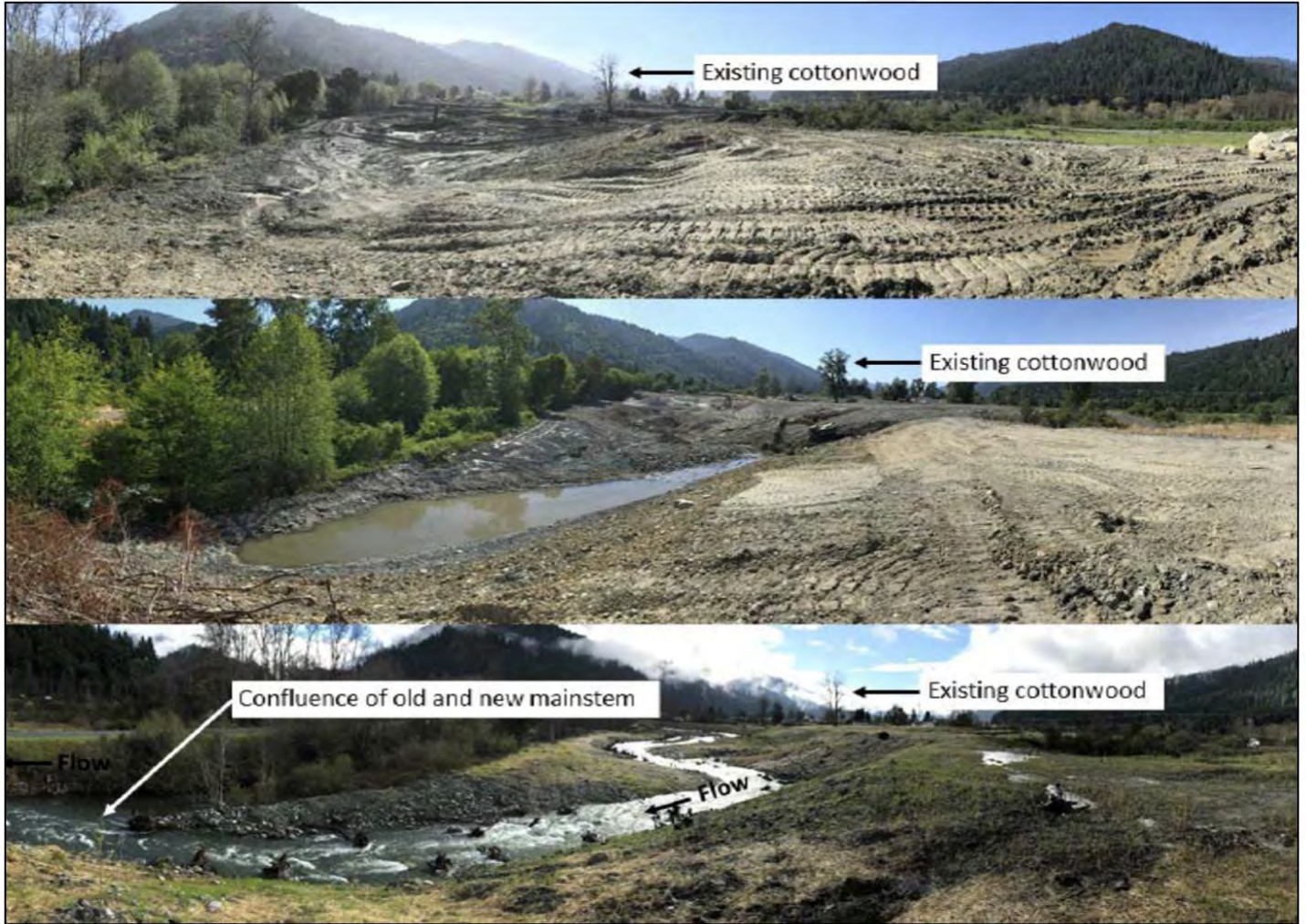
Figure 3. Watershed restoration activities at Mill Creek, during construction (top and middle) and after construction (bottom).
