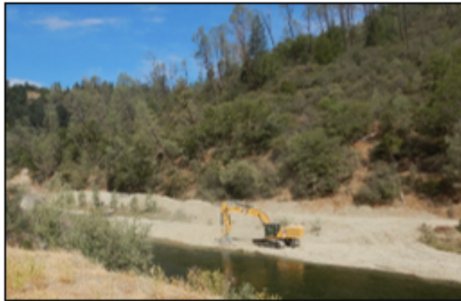
Photo 1. Gravel augmentation near Trinity River Hatchery in summer 2021.
