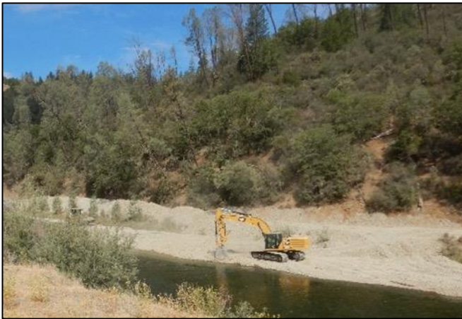
Sediment augmentation near Trinity River Hatchery in Summer 2021 (photo: TRRP)
