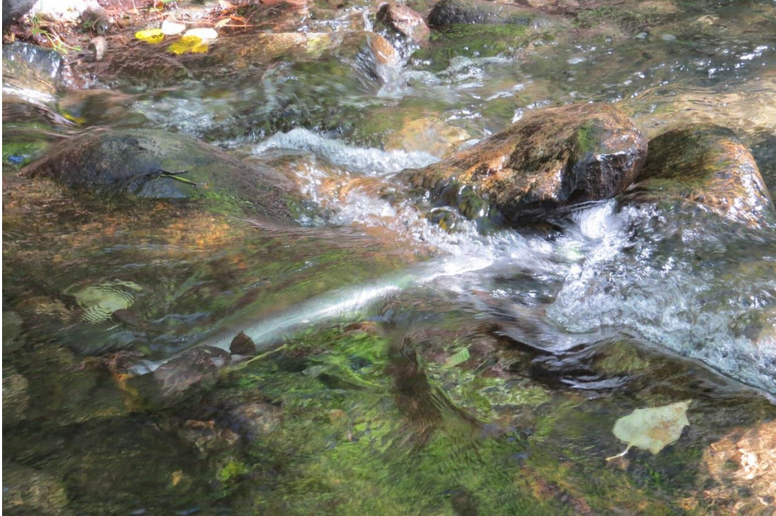
Figure 5: New intake structure equipped with 20 gauge perforated stainless steel screen with 0.075" screen openings and low entrance velocity design to minimize vortices and debris accumulation. This is a non self-cleaning, passive screen with no moving parts to maintain or replace.
