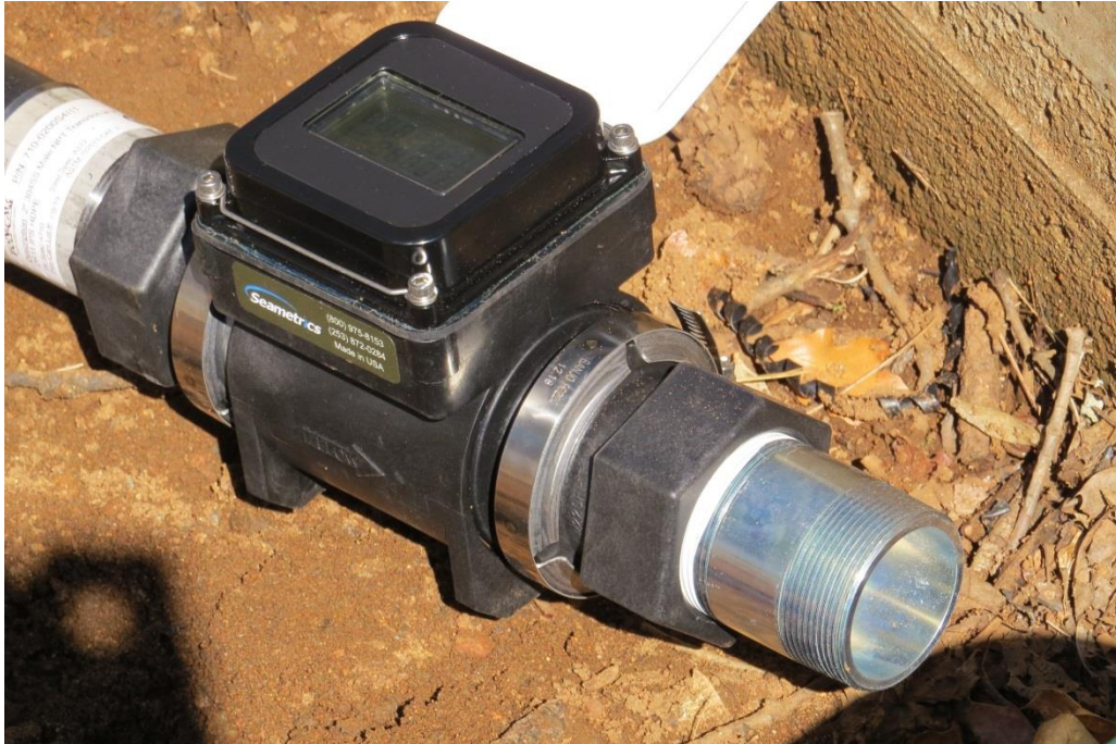
Figure 82: Seametrics Magnetic flow meter (2-inch) and flow regulating Dole valve. Plastic-bodied and battery-powered magmeter irrigation flow meter with digital display functions with no moving parts for unobstructed flow and minimal flow disturbances. Meter allows the user to easily read instantaneous flowrate in GPM and Total volume in gallons. System ensures durable fluid measurement
