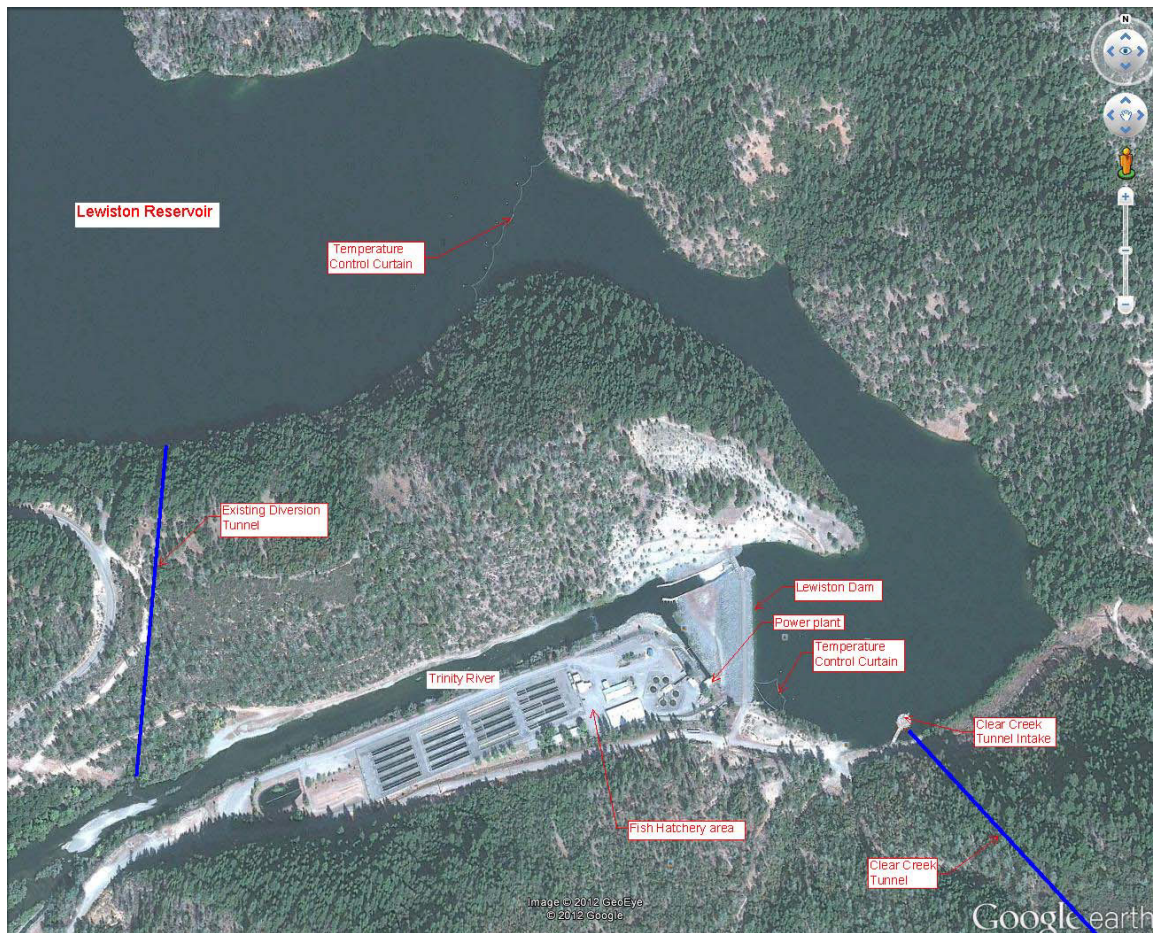
Figure 16. Lewiston Dam and associated points of diversion and other facilities. Figure from USBR (2012). The diversion tunnel on the left (west) side of the image was used during dam construction and is not currently utilized.
