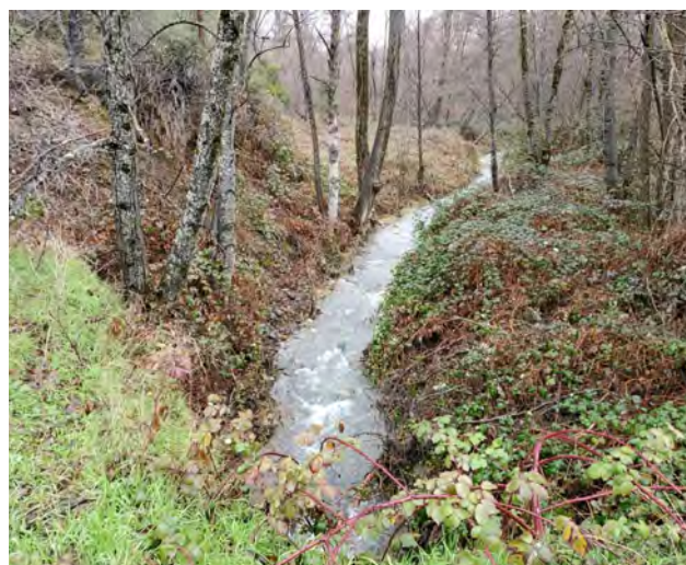
The Yurok Tribe has been awarded funding to design and work through compliance for replacement of the Sky Ranch Road culvert on Oregon Gulch. (Elliot Sarnacki, Reclamation)
