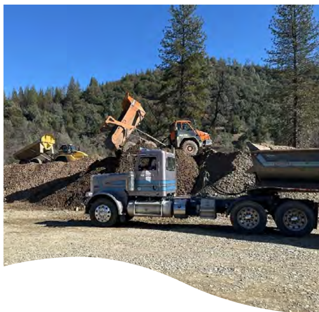
Articulating trucks staging material for haul off to Eagle Rock, Inc. (Elliot Sarnacki, Reclamation)
