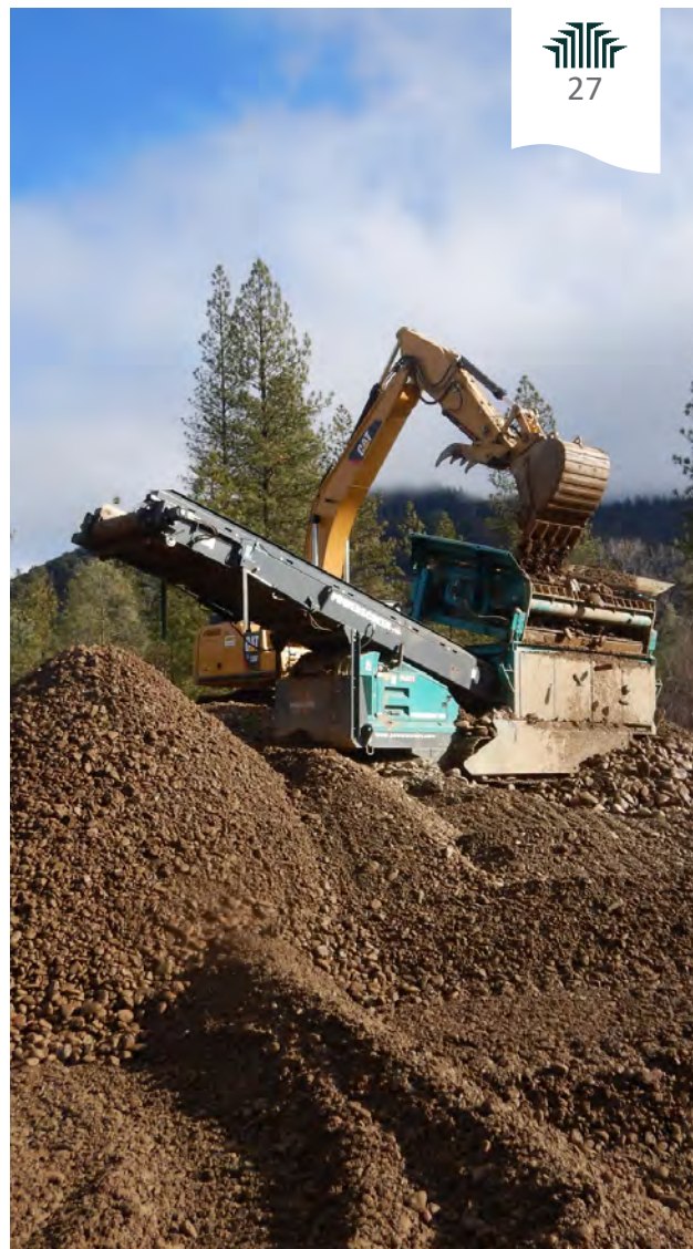
Power screen processing machines sort tailings for building materials and other TRRP project features. (Elliot Sarnacki, Reclamation)
