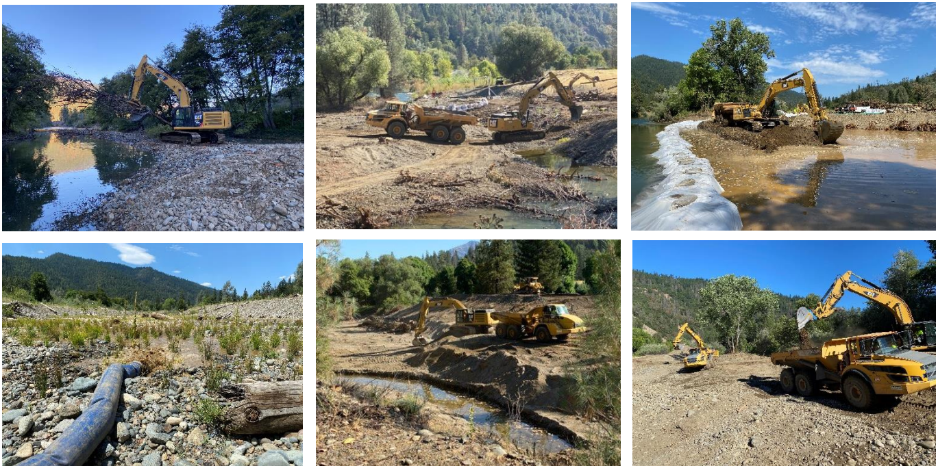
Figure 6. Chapman Ranch Phase B features during construction. (TRRP)
