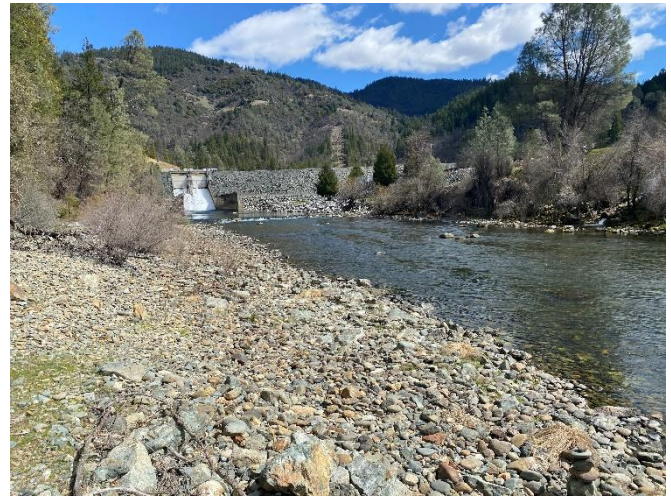
After gravel placement, downriver of Lewiston Dam. (TRRP)
