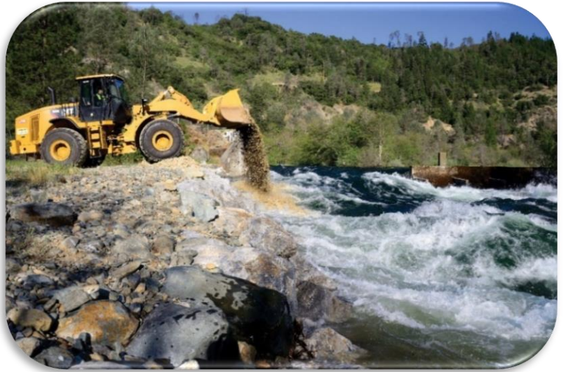
Gravel Augmentation at Lewiston Weir, 2017. (TRRP)
