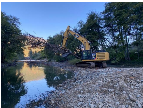
Heavy machinery creates Beaver Dam Analogues (BDAs) to increase wetted areas and provide juvenile fish rearing habitat within the river reach at Chapman Ranch restoration site, 2021. (TRRP)
