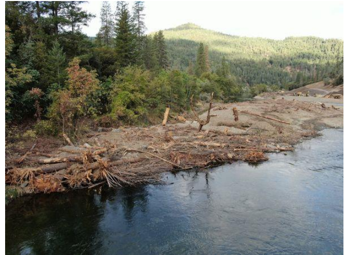
A large wood instillation at Dutch Creek Restoration Site completed in 2020. (TRRP)
