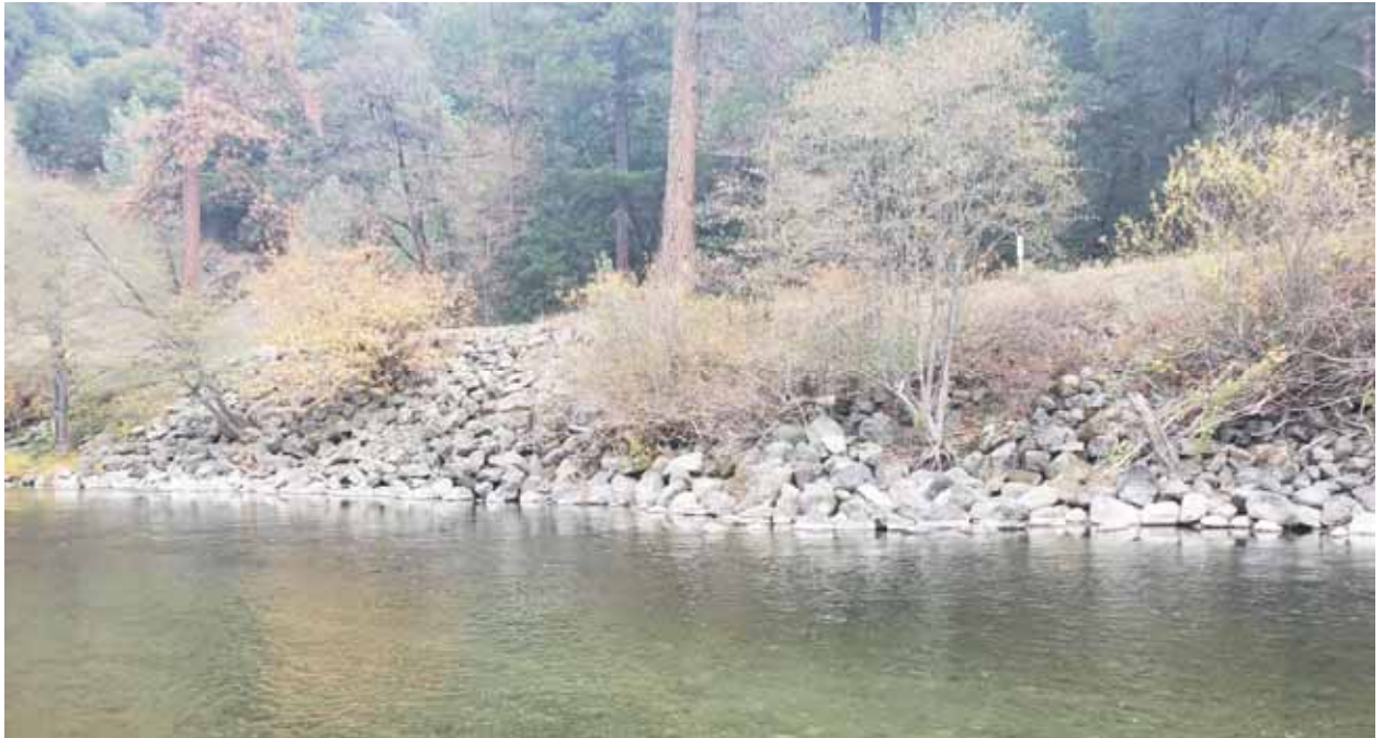
Figure 5. Riprap along the right bank from RM 77.5 to RM 77.8.
