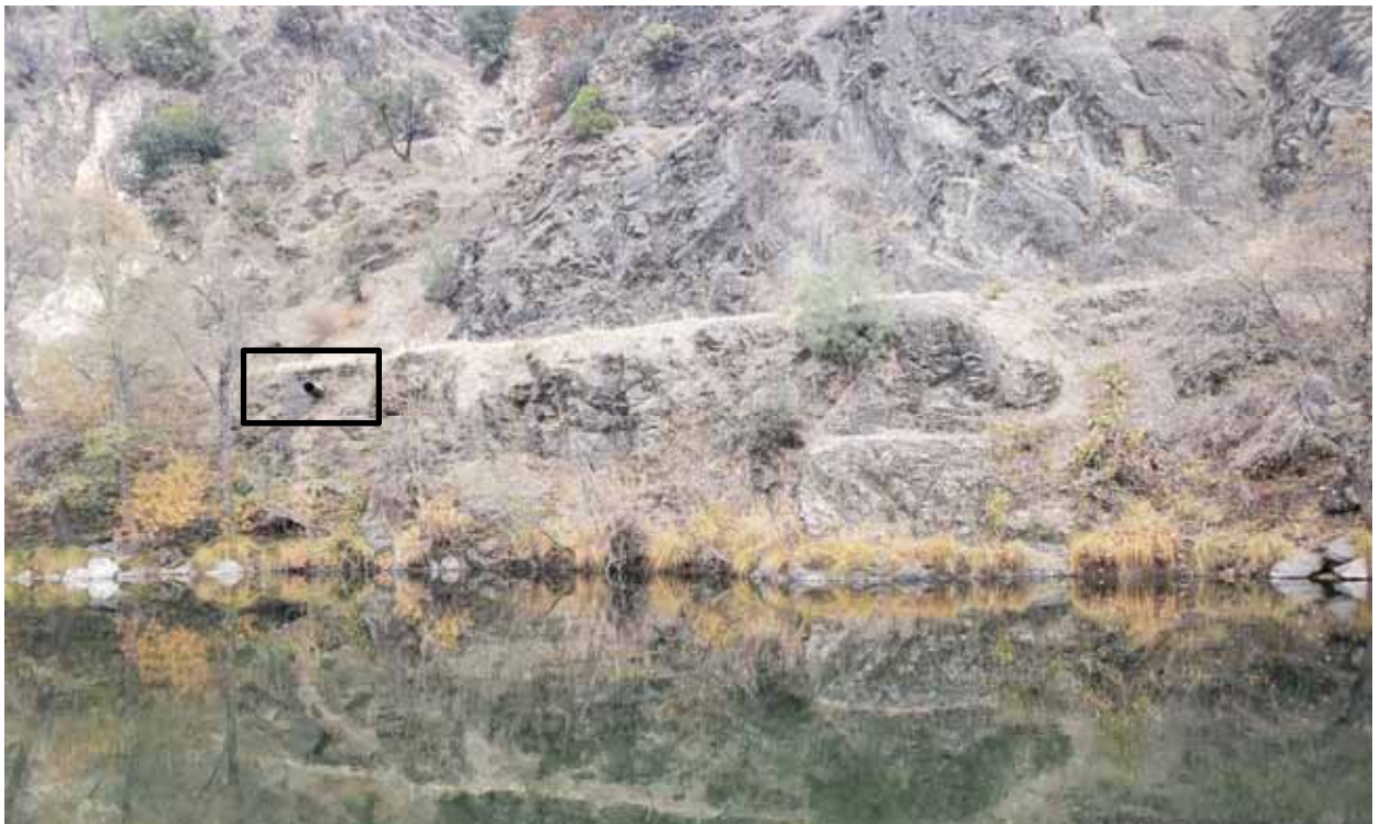
Figure 6. Existing wall with culvert used for Highway 299 drainage (outlined in black).
