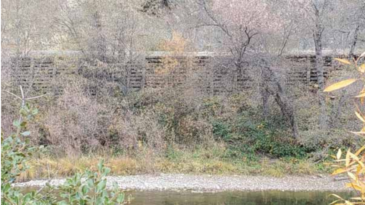
Figure 7. Concrete crib wall on river right along Highway 299.
