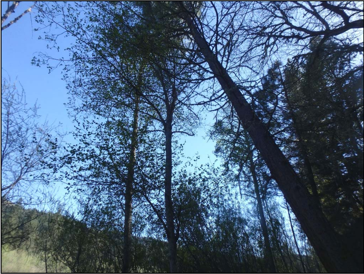
Figure 18. Photograph of TRGV sampling cableway anchor leaning toward mid-channel. View is downstream.
