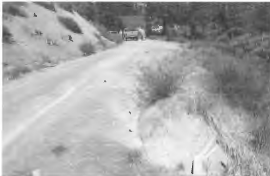
Figures L and M. Pre implementation conditions on road 31N38 included failed overside drains.
