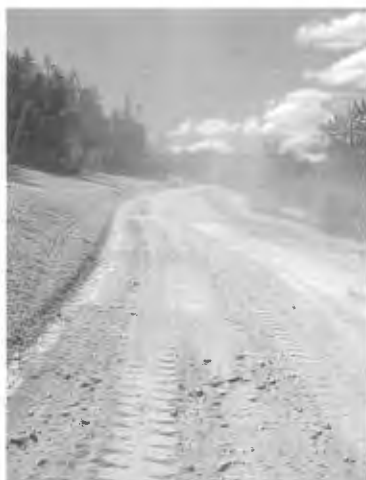
Figure B. Blading/shaping that was performed on road 1S23.
