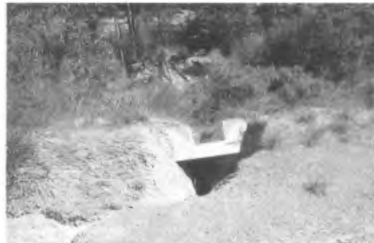
Figures L and M. Pre implementation conditions on road 31N38 included failed overside drains.
