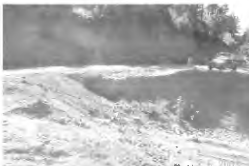
Figures H and I. . Pre and post implementation photos showing re-shaping unstable road fill slope on Road 4N24, MP 3.03
