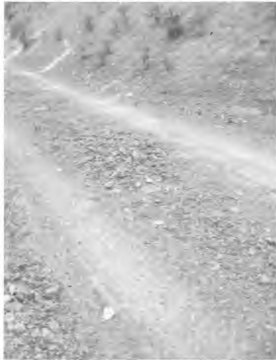
Figure O. Photo of rockered roadway on road 31N38.
