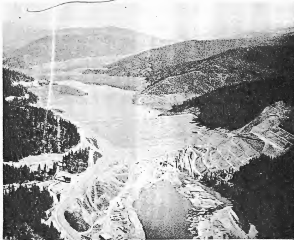
Trinity Reservoir Takes Shape Behind the Dam
