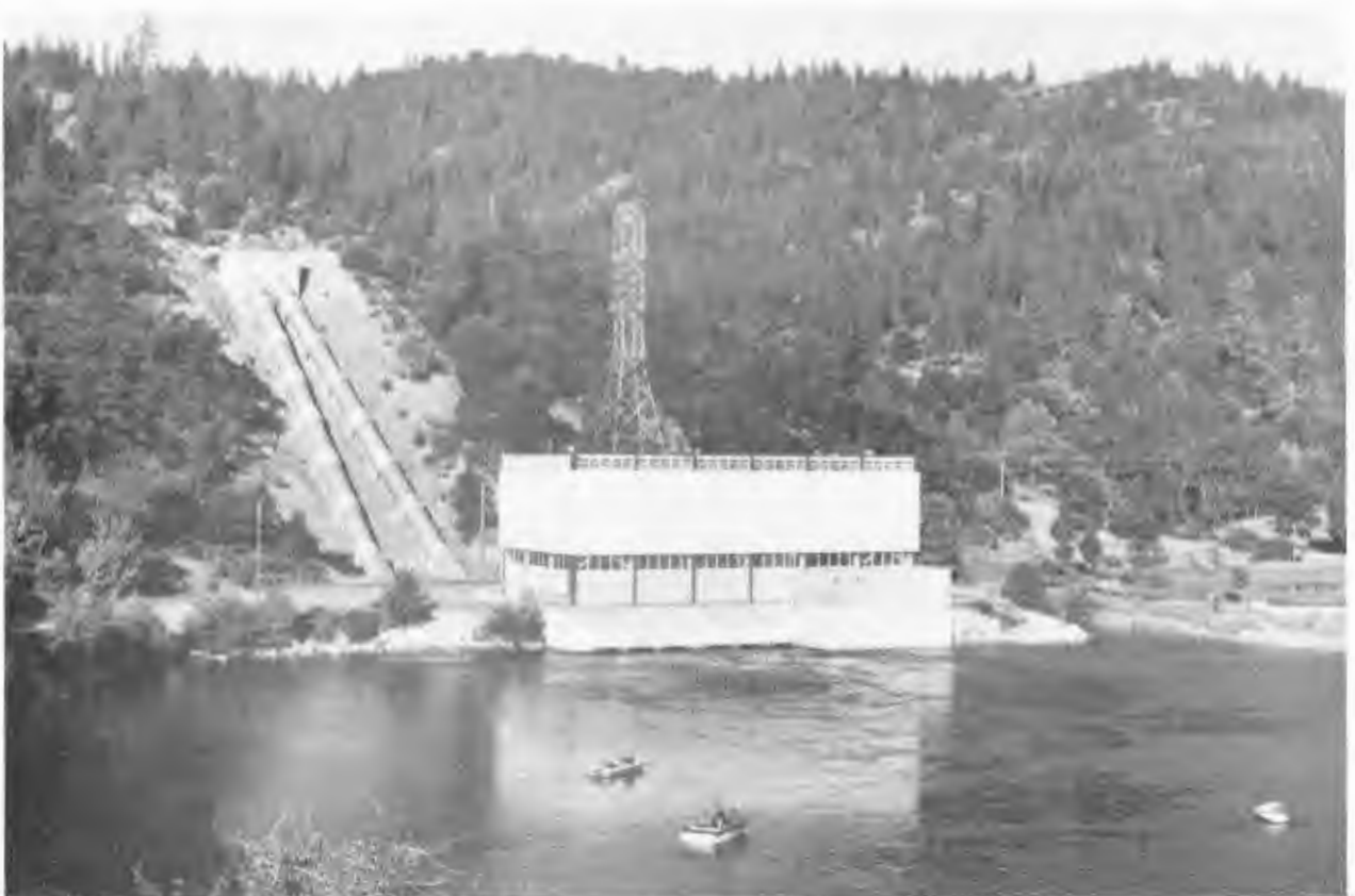
General view of the penstocks carrying water to the Judge Francis Carr Powerhouse from the Trinity River. The body of water in the foreground is part of Whiskeytown Lake.
