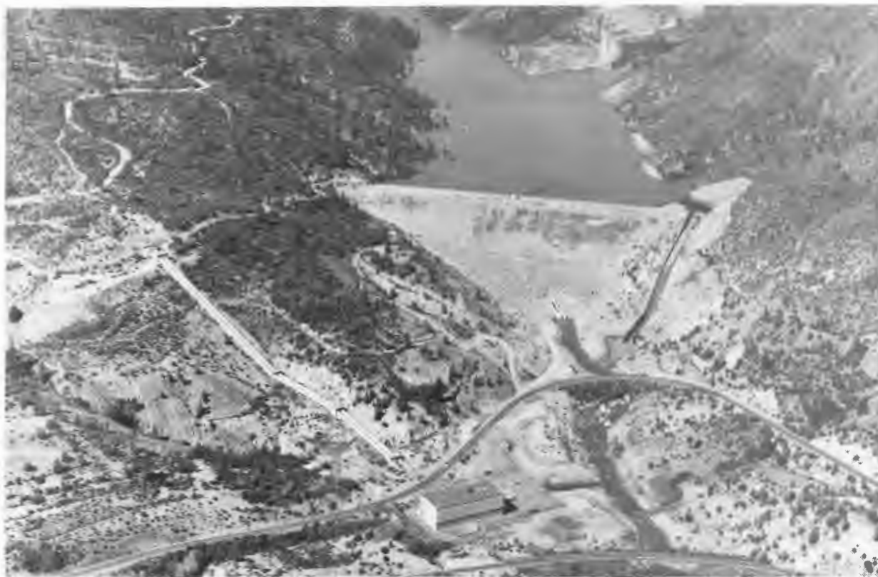
Aerial view of the Spring Creek Debris Dam (background) and the Spring Creek Penstocks and Powerplant in the foreground. Water from Whiskeytown Lake is diverted by the Spring Creek Tunnel and Powerplant to Keswick Reservoir.
