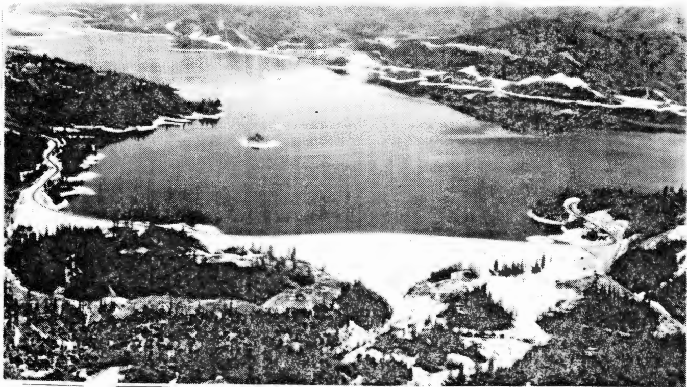
Aerial view upstream of Whiskeytown Dam and Lake. Note vehicular road traversing the earthfill dam across the lower central area of the photograph.
